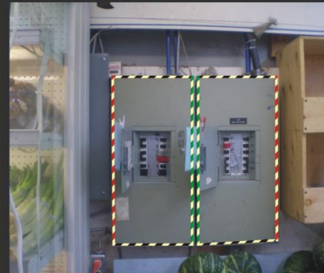
Self Adhesive Photoluminescent Tapes used as edge markers around the electrical panel
